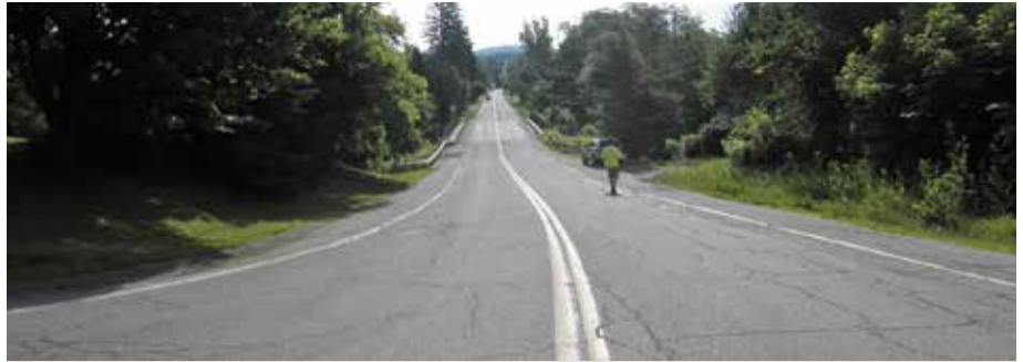
POST MILLS. Cracked pavement on VT 244.
