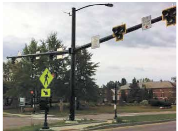
COLCHESTER. After construction, view of new HAWK signal looking toward Fanny Allen.
