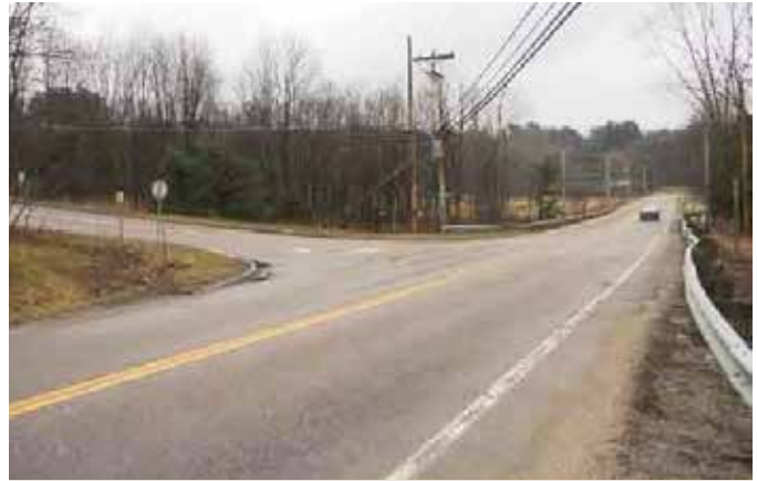
ESSEX TOWN. Looking east, along VT 117 with Sand Hill Road on the left before construction.
