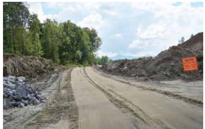
MORRISTOWN. View of blasting area north of Bridge Street.
