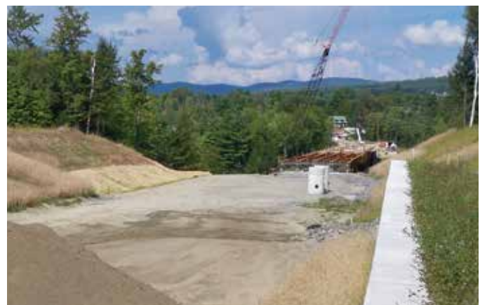
MORRISTOWN. View of mechanically stabilized earth wall at southern bridge approach.
