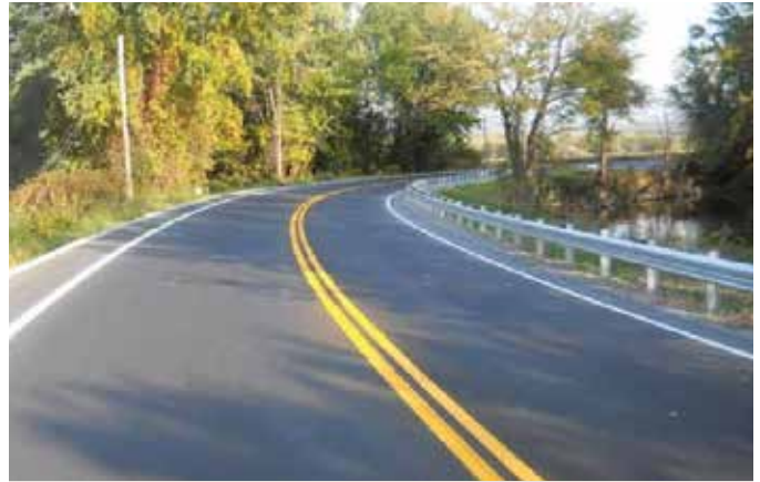
SUDBURY. New reclaimed roadway and guardrail abutting Otter Creek.
