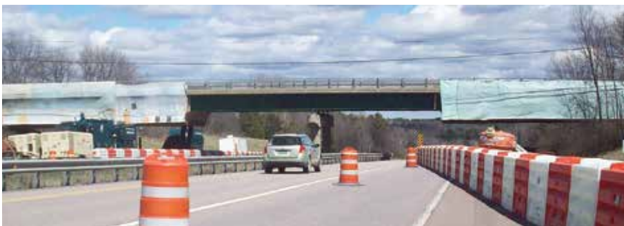
MILTON. A bridge over I-89 tented for painting. By removing aging lead paint and replacing it with an advanced polymer coating, we simultaneously extend the life of the structure and eliminate an environmental hazard.
