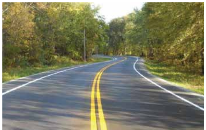
SUDBURY. Significant grade increase where most severe flooding occurred.
