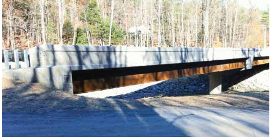
JAMAICA. This bridge on VT 100 utilized accelerated project delivery, moving from survey to contract plans in only 11 months.
