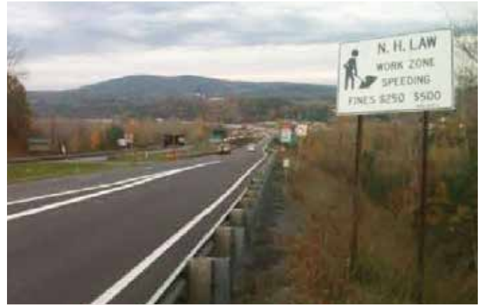
HARTFORD. I-89 Southbound Lane, looking south into New Hampshire.
