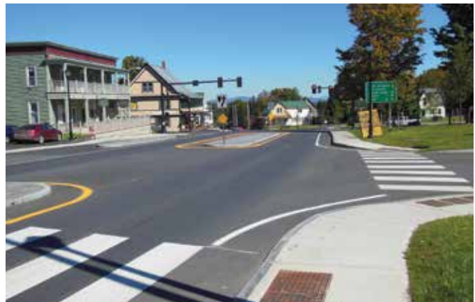
DANVILLE. Looking east on US 2 in the village.
