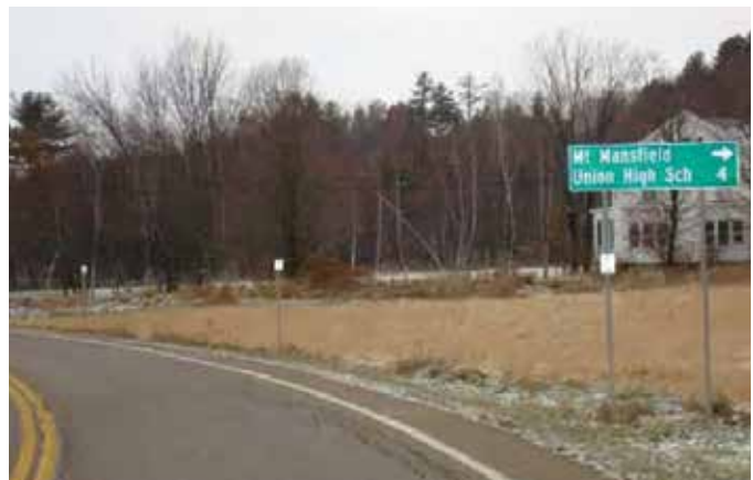
JERICO. Project after improvements which included installation of new 6"x 8" rectangular white delineators.
