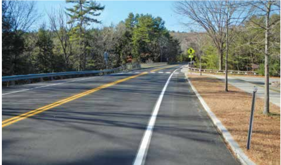
HARTFORD. Approaching Quechee Gorge on VT 4. Centerline rumble stripes were one of many safety improvements made in partnership with the Vermont Highway Safety Alliance.
