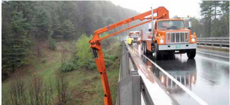
WINDSOR. A bridge inspection team utilizes a service lift on I-91.
