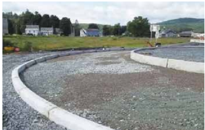
CAMBRIDGE. During construction, looking west along VT 15 across the truck apron. The central island is on the right.
