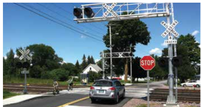
ST. ALBANS. Newly completed crossing upgrade.
