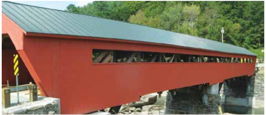
WOODSTOCK. The Taftsville covered bridge was completely restored after being severely damaged by Tropical Storm Irene.
