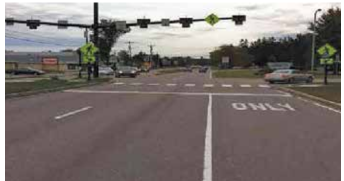
COLCHESTER. After construction, looking easterly along VT 15 towards Essex.
