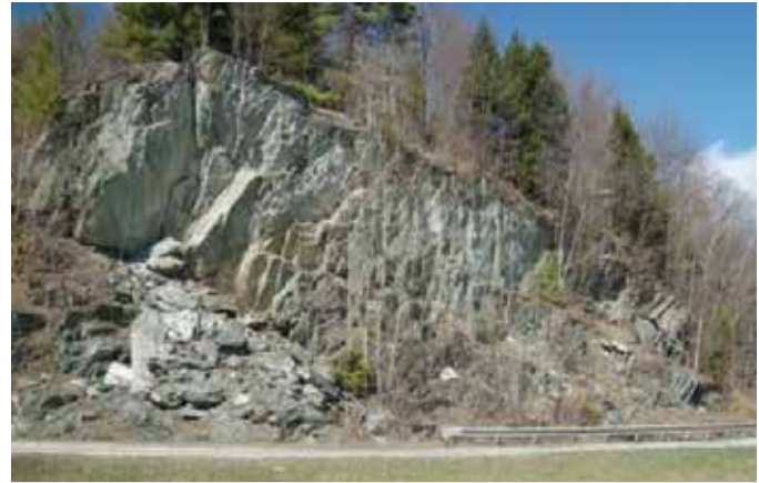
MONTPELIER. Prior to construction. Ramp B ledge cut.
