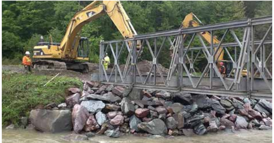
WESTFORD. VTrans Operations' Statewide Bridge Crew works to install a temporary bridge on Seymour Road in Westford. A dozen families were stranded due to the washout of the town road during the summer 2013 marathon of thunderstorms.
