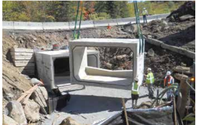
SEARSBURG. Phase II pre-cast box culvert section installation.
