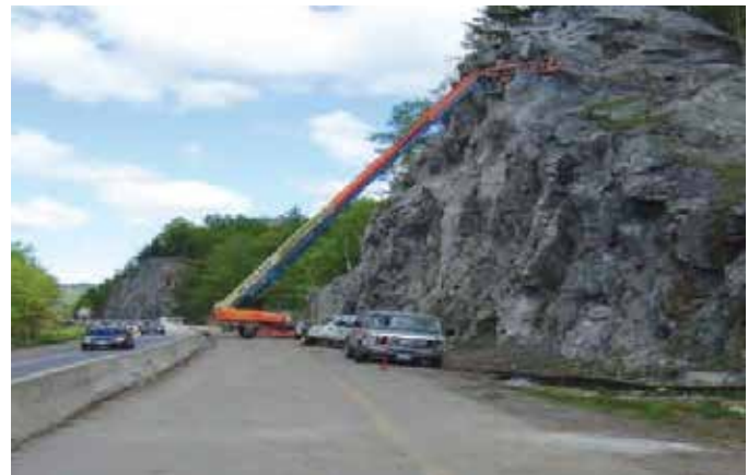
RICHMOND. During construction.
