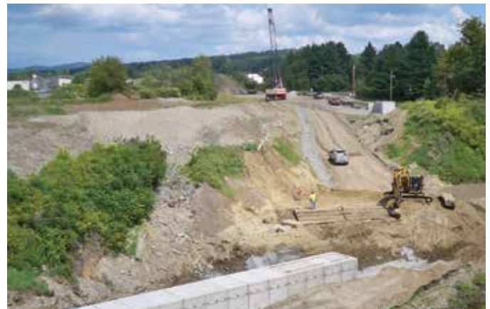
MORRISTOWN. During construction of the ravine culvert.
