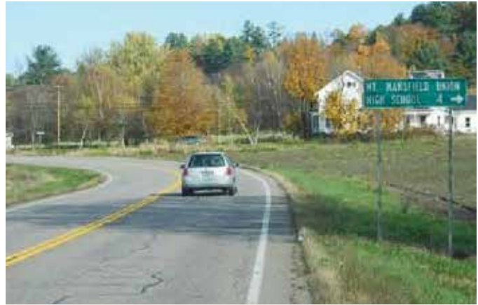
JERICO. HSIP Example Project Site in Jericho on VT 117 near Barber Farm Road intersection. Picture was taken before safety improvements. Note the lack of delineation around the curve.
