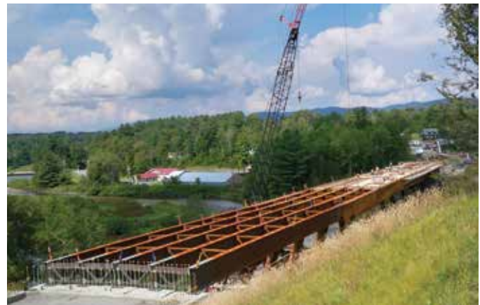
MORRISTOWN. View of the top of the bridge looking north.
