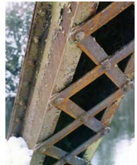
BARNET, VT/MONROE, NH. Lacing on a truss member.
