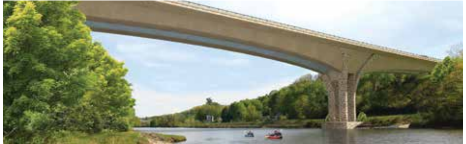
BRATTLEBORO. Spanning VT 30 and the West River, this design/build project is currently under construction on I-91 and will replace two aging bridges with a single span.
