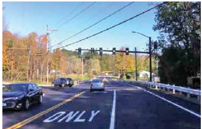
ESSEX TOWN. Looking east, along VT 117 with Sand Hill Road on the left, after signal, pavement and line striping installation.
