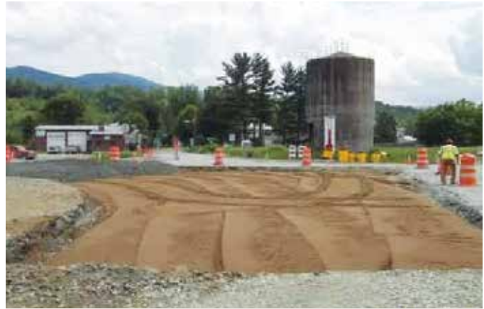
CAMBRIDGE. During construction, looking southerly across the intersection.
