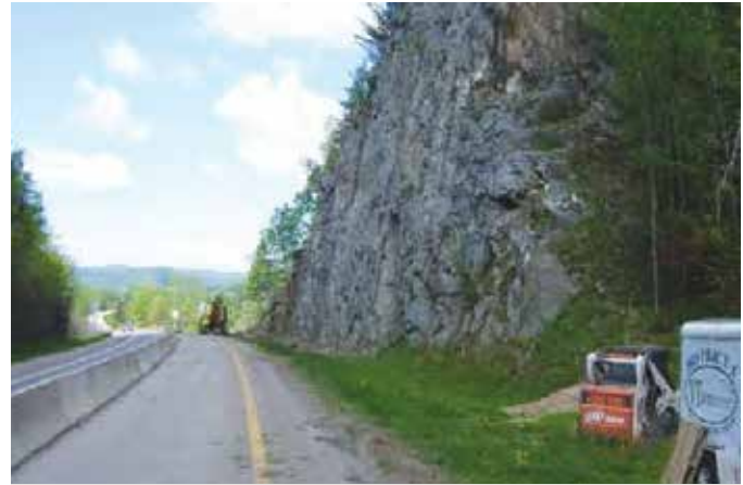
RICHMOND. During construction.
