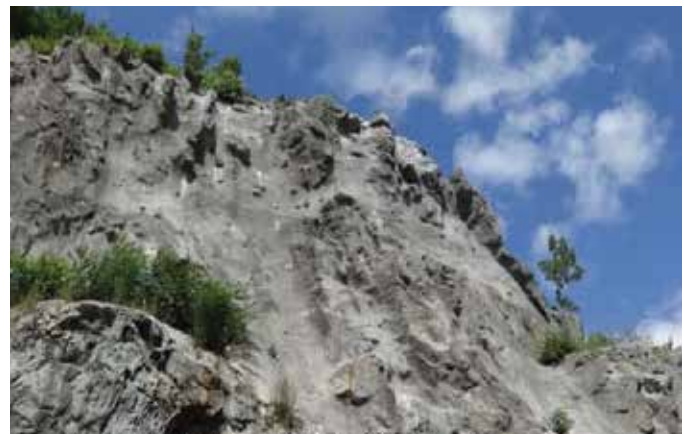
RICHMOND. After construction.
