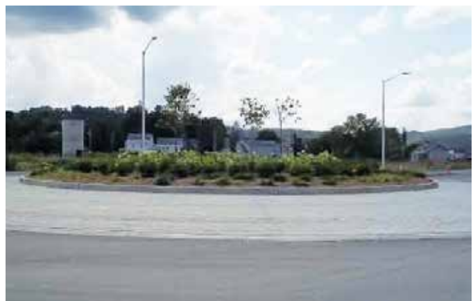
CAMBRIDGE. After construction, looking west down VT 15, from the eastern splitter island.
