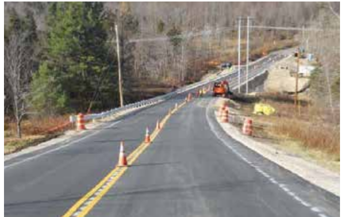
SEARSBURG. Completed culvert installation and roadway reconstruction.
