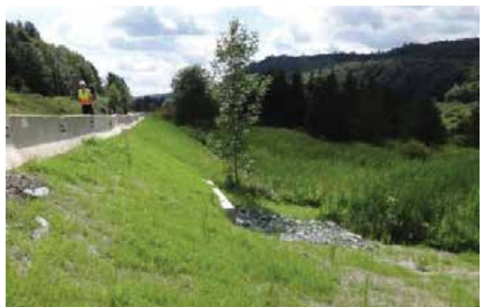
FLETCHER. Northern slide during construction, looking south along VT 108.
