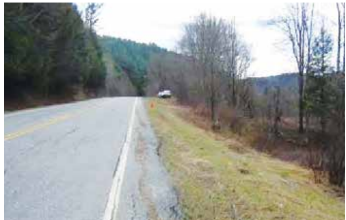
FLETCHER. Southern slide before construction, looking south along VT 108.
