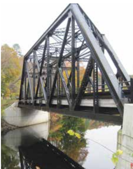
SPRINGFIELD. Rehabilitated truss bridge.
