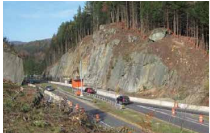
MONTPELIER. During construction. Ramp A and Montpelier State Highway ledge cut.
