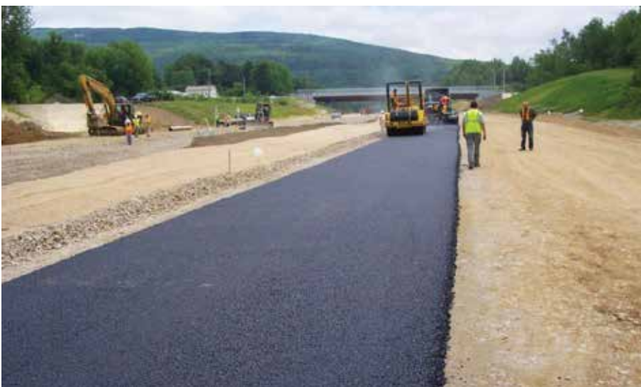
BENNINGTON. US 279. An example of engineered pavement.
