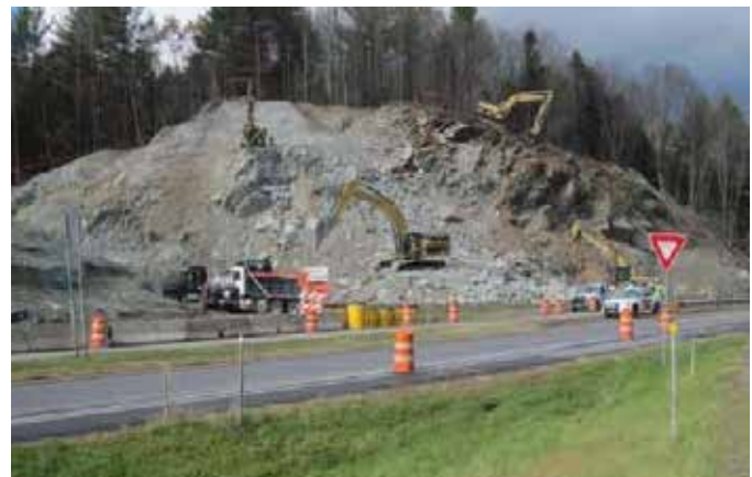
MONTPELIER. During construction. Ramp B ledge cut.
