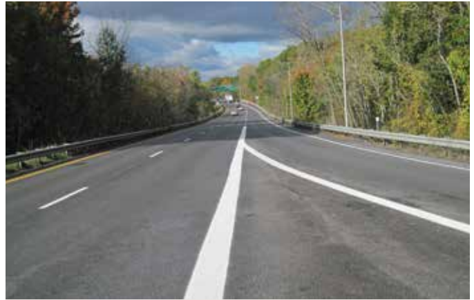
BENNINGTON. Newly installed pavement markings on US 279.
