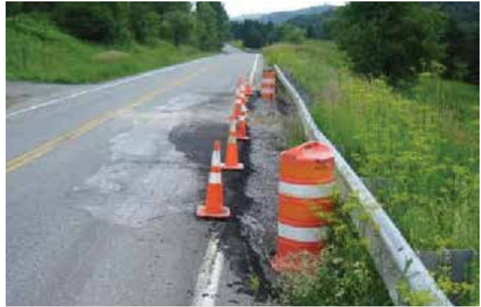
FLETCHER. Northern slide before construction, looking south along VT 108.
