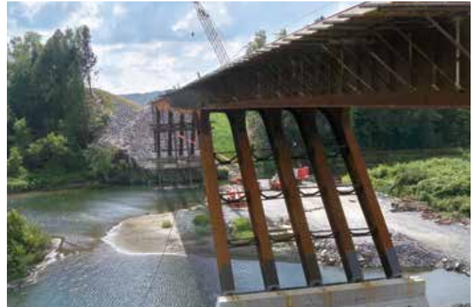
MORRISTOWN. View of bridge looking south.
