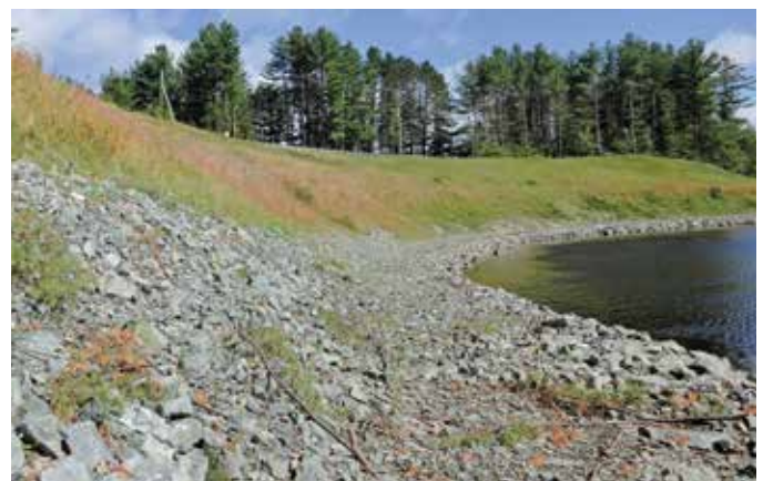
MAIDSTONE. Prior to construction. Slope adjacent to VT 102.
