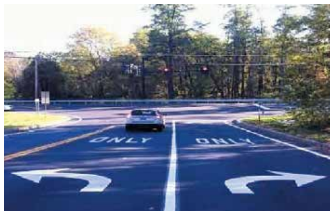
ESSEX TOWN. After completion, looking at the intersection from Sand Hill Road.
